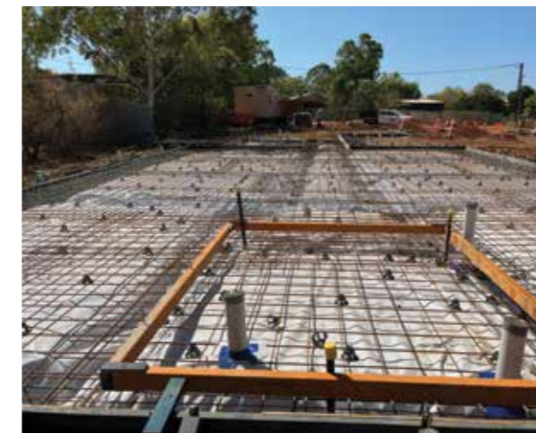
Lajamanu - 8 bedroom, 3 bathroom staff house
