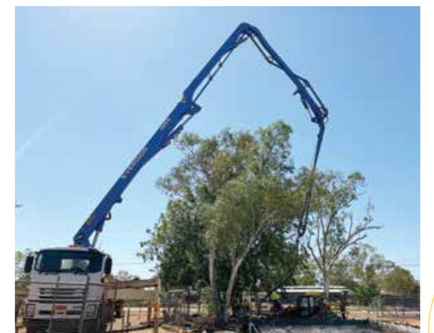
Kalkaringi - 6 bedroom, 2 bathroom staff house
